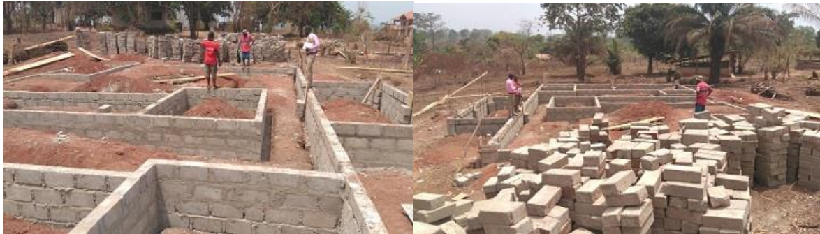
Beginning of works
