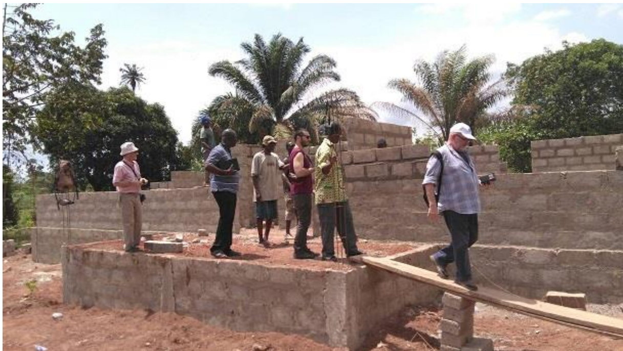
Inspection of the on-going Laboratory and Pharmacy
