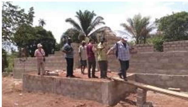
Inspection of the on-going Laboratory and Pharmacy Project at Oseikojokrom
