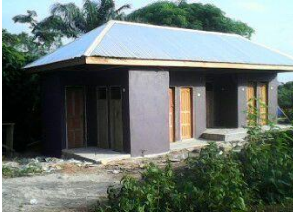
The new washroom at St. John of God Clinic, Oseikojokrom
