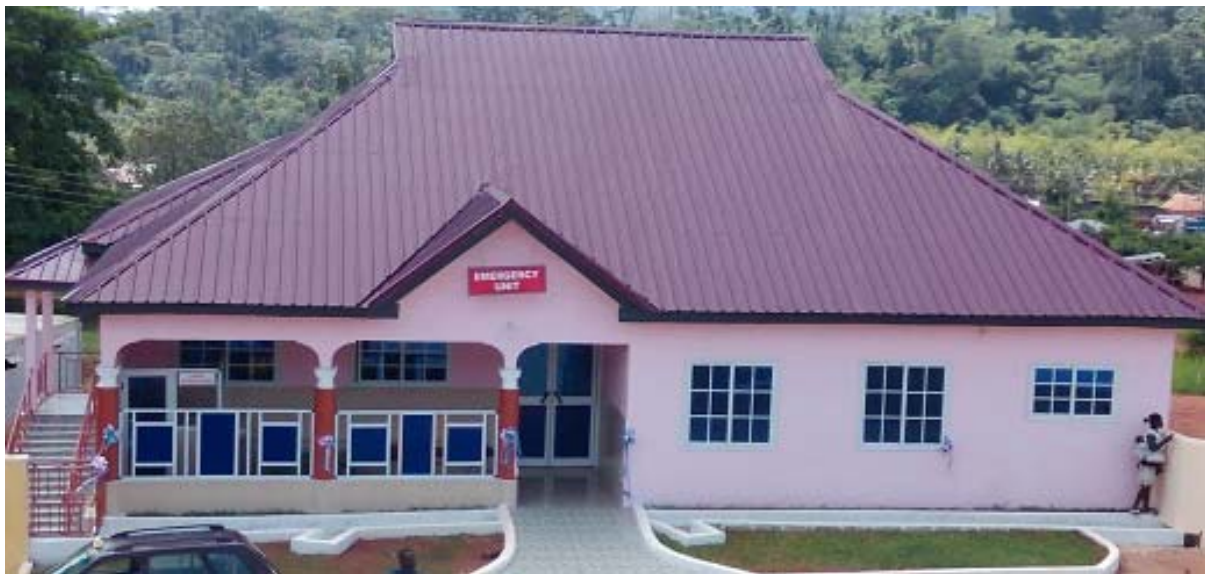
FRONT VIEW OF THE NEW EMERGENCY BUILDING
